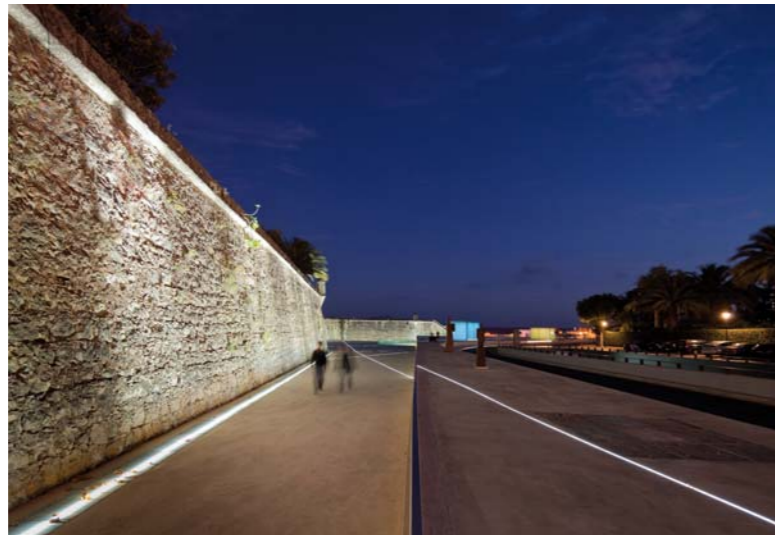
The 'Praça Diogo de Meneses' in Caiscais, Portugal presents all operational lighting restricted to the vertical surfaces of the fort wall. Replicating ancient Portuguese sailing charts, the linear recessed feature lighting provides guidance and direction to the users. There are no columns within the entire square. Short-listed for the Mies Van Der Rohe 2011 Award. Lighting design: Miguel Arruda Arquitectos Associados in cooperation with Donker - Light Glass Technology". Photos: Miguel Arruda Arquitectos Associados.
